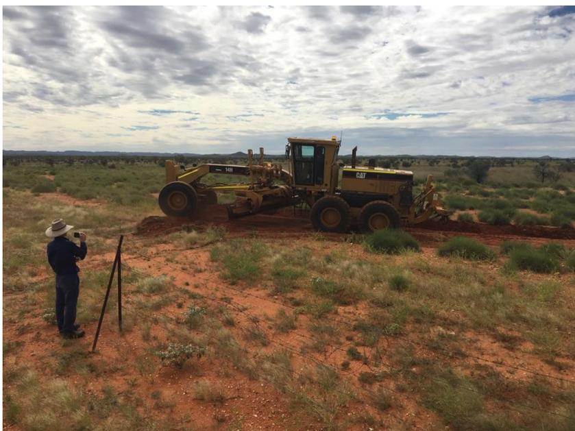
Darryl Hill operating Limestone Station's grader, demonstrating earth bank design and construction to Grant Brooks, while Grant videos the demonstration to refer back to later.
